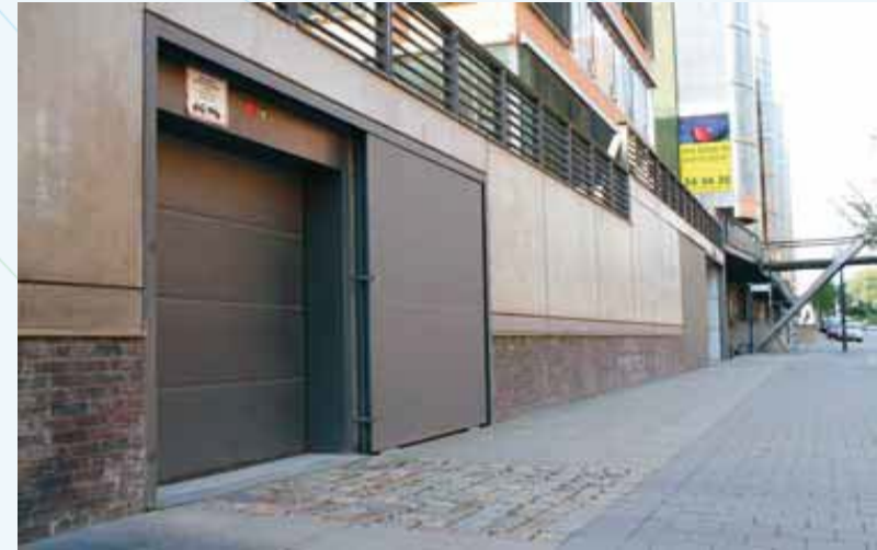
Example of adaptive building (flood door)
